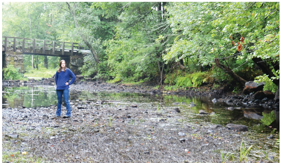
Winthrop Bridge over the Ipswich River, September 2016 . Photos by Suzanne Sullivan.
