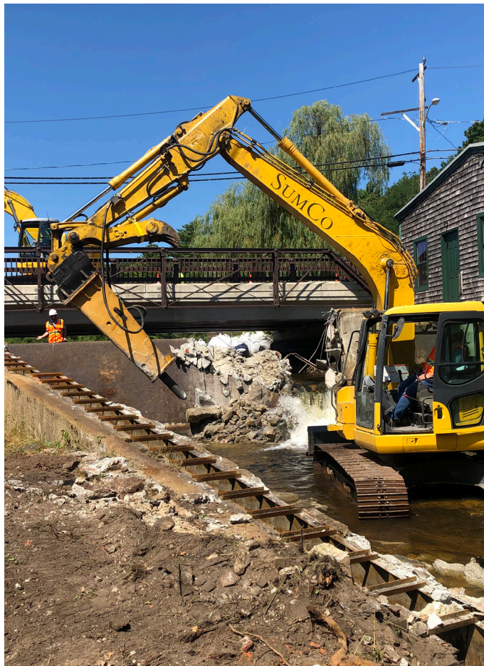
Elm Street Dam Removal in Kingston, MA
