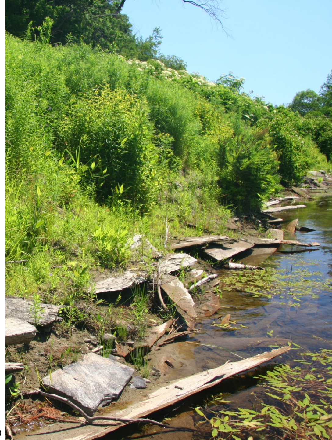
Cut logs eroding out of the left bank, upstream of Head Tide Dam, Sheepscot River, Maine (July 2016)
