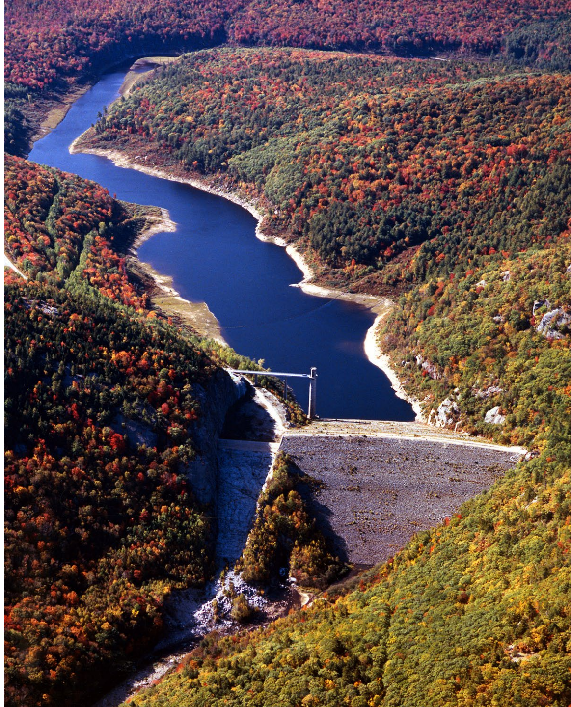
Flood control dam: Ball Mountain Lake, West River, VT (USACE, 1999)
