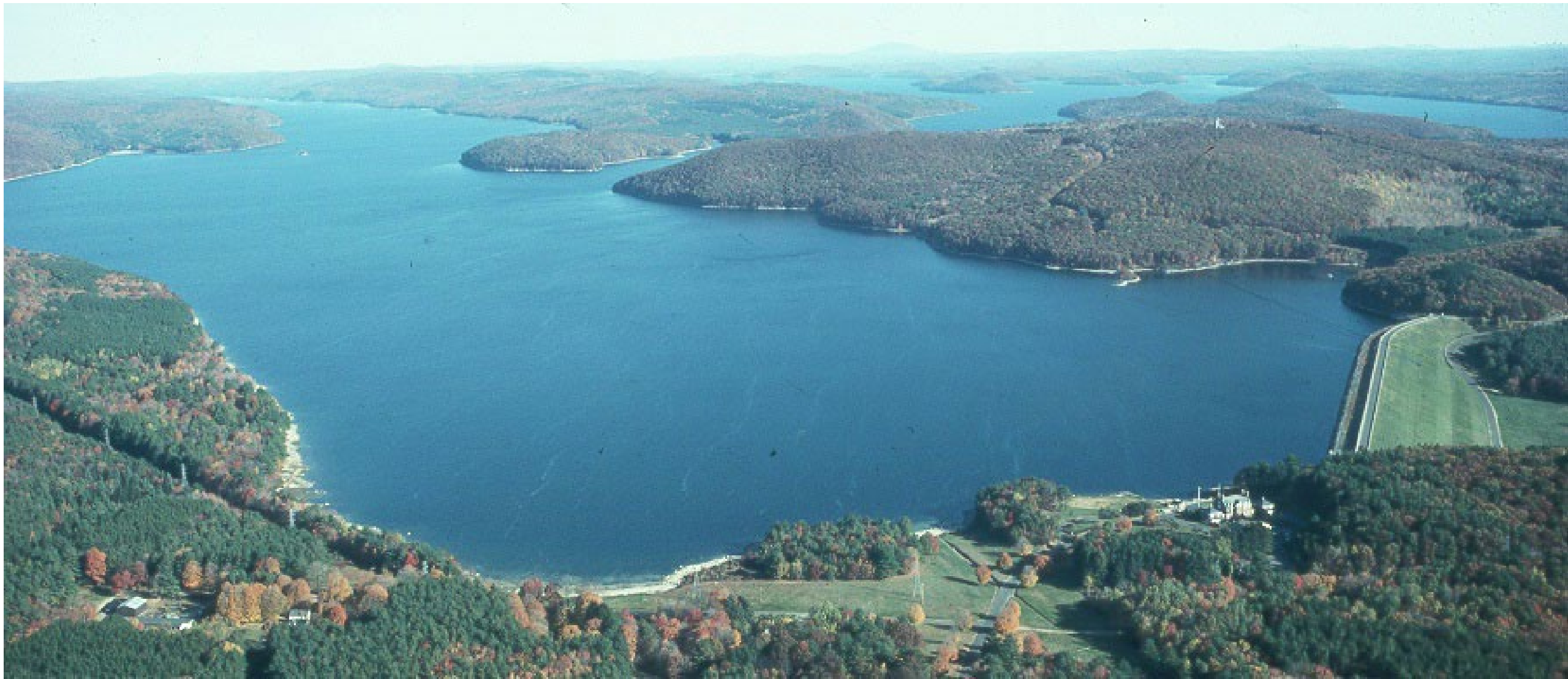
Quabbin Reservoir and Winsor Dam, Swift River, MA, 1946 (massmoments.org) 170 ft (52 m) high, 412 billion gallons of water storage (1.56 km 3 )
