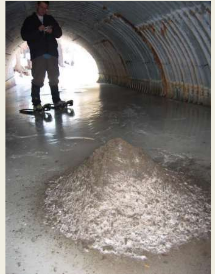
Roadway sand and salt pile underneath a storm drain and on a frozen stream
