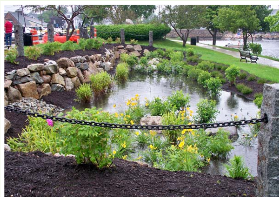
Constructed wetland intercepting urban drainage in Plymouth, MA. Photo courtesy of Horsley Witten Group.
