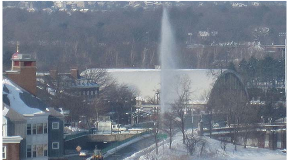
Broken water main (installed in 1914) on Soldiers Field Road in Cambridge, 2011. Photo Courtesy of Massachusetts Water Resources Authority.
