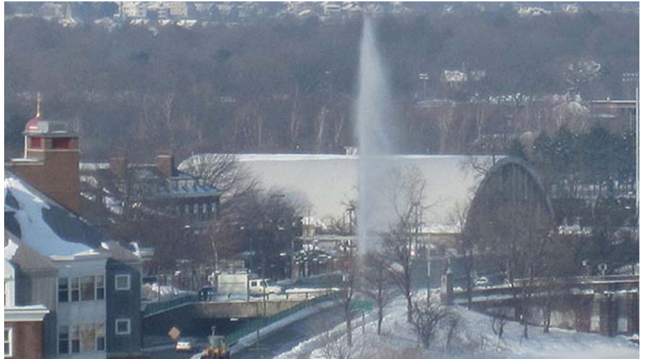
Broken water main (installed in 1914) on Soldiers Field Road in Cambridge, 2011. Photo Courtesy of Massachusetts Water Resources Authority.
